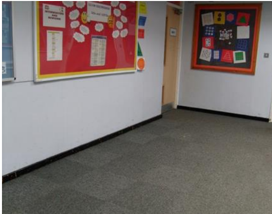
Picture 3 – Student taken photograph of floor and seating area
