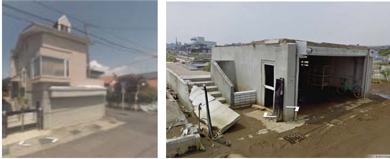
Figure 10 Dual frame construction building A25 in Ishinomaki ‘Before’ (GSV, 2013d) (left) and ‘After’ (GSV, 2013c) (right)
