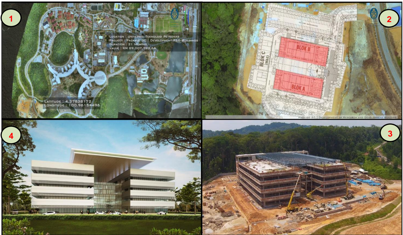
Figure 1 Construction site, UTP R&D
