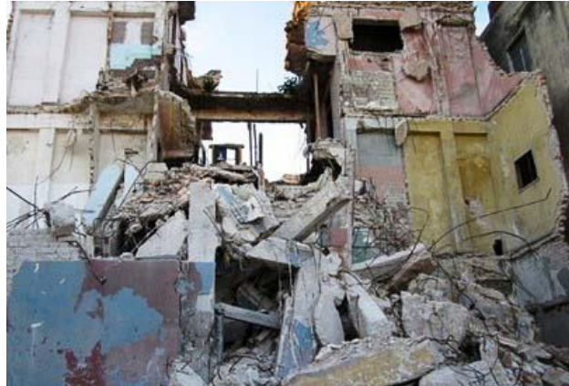
Figure 1. Demolition waste of a building in Havana, where the mixing of different materials can be observed. Source: self-elaboration.
