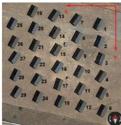
Figure 4.5. Dual-axis trackers plant Peñarroya I
