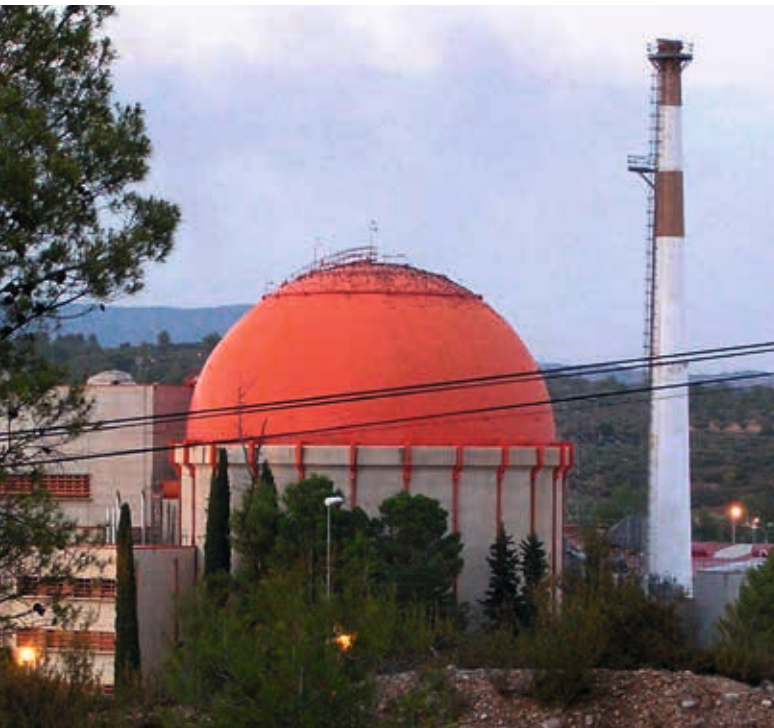
Picture of the José Cabrera nuclear plant in Almonacid de Zorita, Guadalajara. It was the first plant of this type in Spain and worked until 2006, when it ceased its activity.
