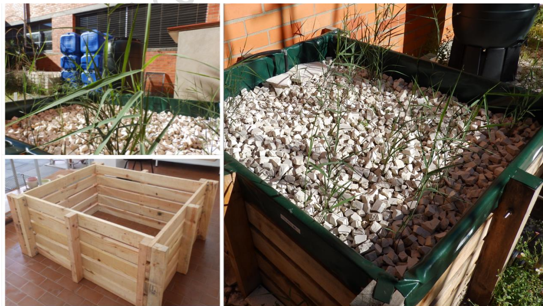
Figure 3 – Pictures of a modular wood-based CW. One of the inserted images shows the wood-based structure.
