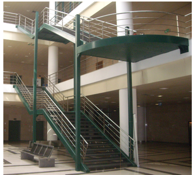
Fig. 1. Studied steel staircase.
