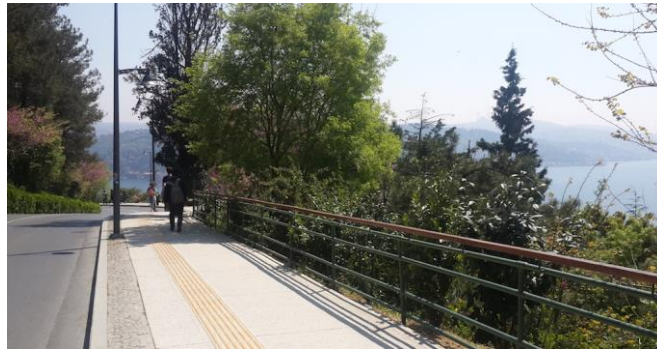
b) Road that connect different offices and student's dormitories.
