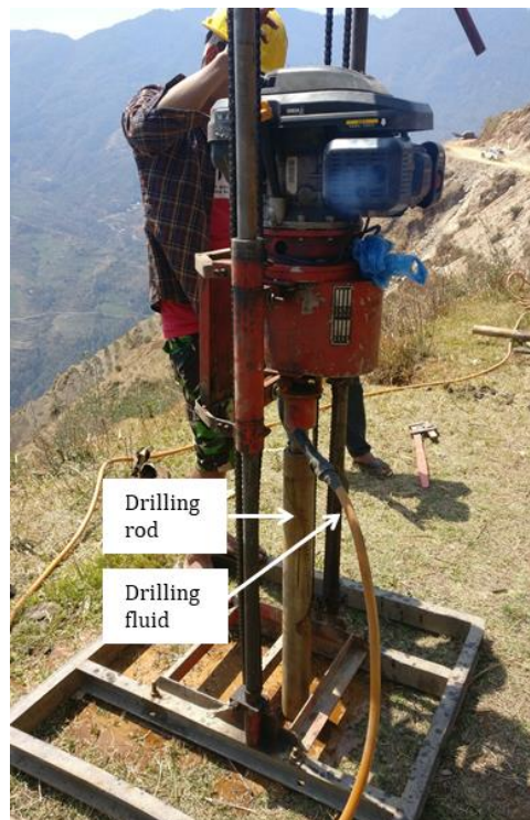
Figure 3.3 Photograph of rotary drilling equipment used in this study.
