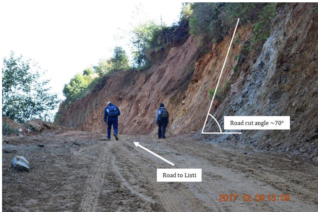
Figure 2.8 Steep road cut along Daklang-Listi road ( 27^{\circ}53'11.1''\text{N} 85^{\circ}53'25.4''\text{E} ).
