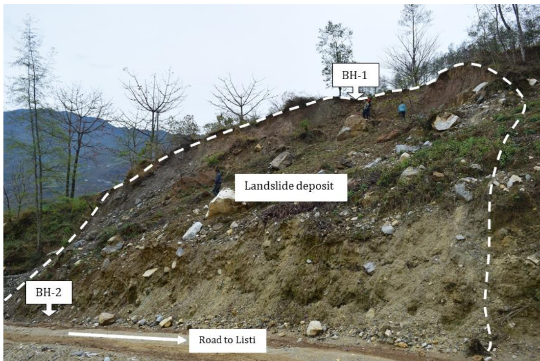
Figure 3.4 Photograph of Kanglang landslide showing the approximate location of boreholes (BH-1 and BH-2).
