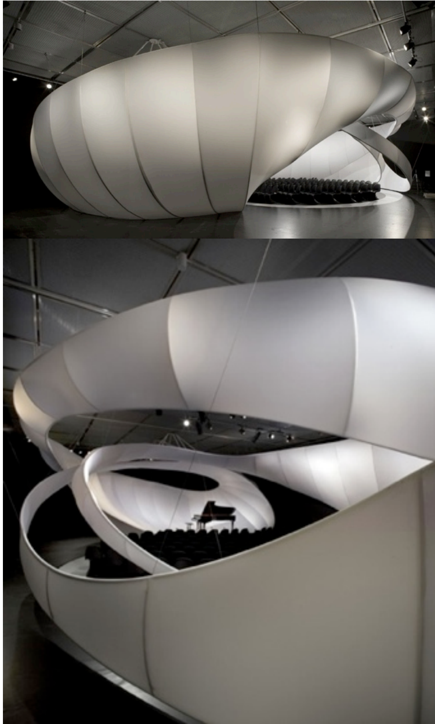
Figure 2-10: Zaha Hadid, the Chamber Music Hall (Manchester International Festival), textiles stretched over a steel structure, 2009. Image source: Zaha Hadid Architects (2009) (internet source).
