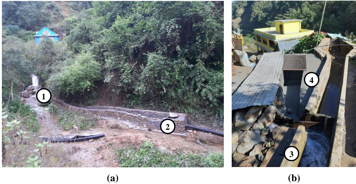
Figure 7.16 - (a) de-silting bay and (b) forebay tank at the pilot site. Numbered labels indicate: 1 – intake, 2 – de-silting bay, 3 – canal, and 4 – forebay tank. Photo credit, Prem Karki.
