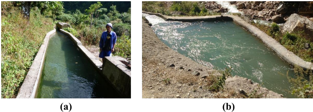
Figure 4.5 – Examples of (a) effective and (b) ineffective forms of de-silting bay. Photo credit, author.
