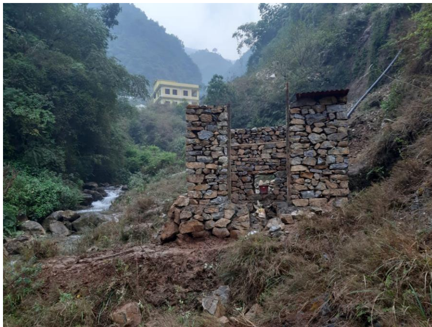
Figure 7.17 - Powerhouse under construction at the pilot site. Photo credit, Prem Karki.
