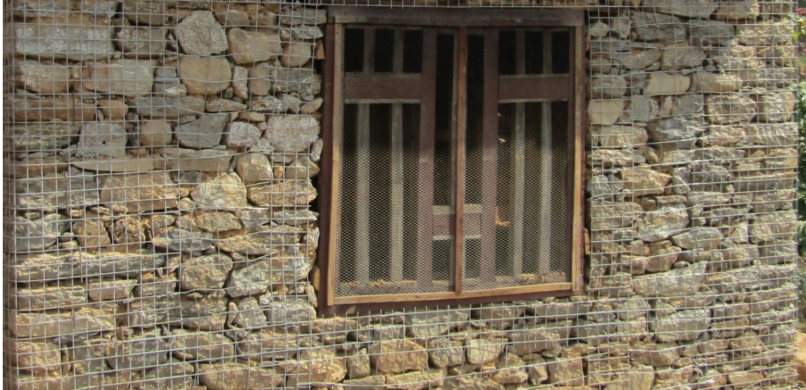
Figure 1 A house with WWM laid over and ready for plaster
