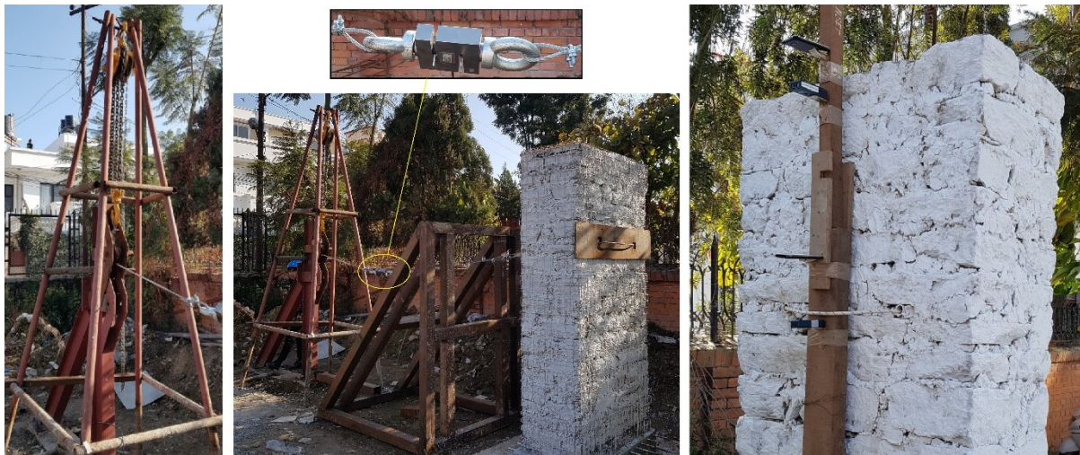
Figure 9 Chain pulley arrangement (left); Pulldown setup for retrofitted wall (mid); Lasers placed pointing towards the retrofitted wall, using the unreinforced wall as support (right)
