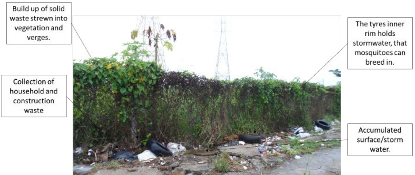
Figure 3-5: Blocked drain nearby favela community. (Photo shared with the author by Participant 5).
