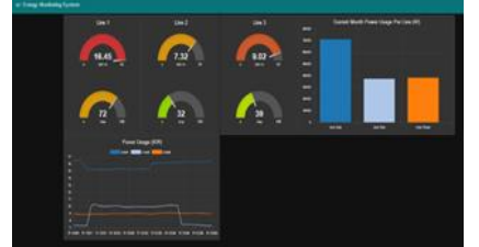
Figure 5: Continuous energy monitoring using our designed system.
