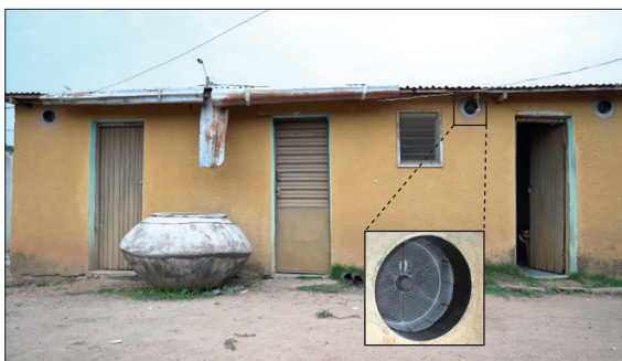
Figure 1: A house in Côte d'Ivoire with screening plus Eave Tubes The inset shows the Eave Tube insert placed within the tube.
