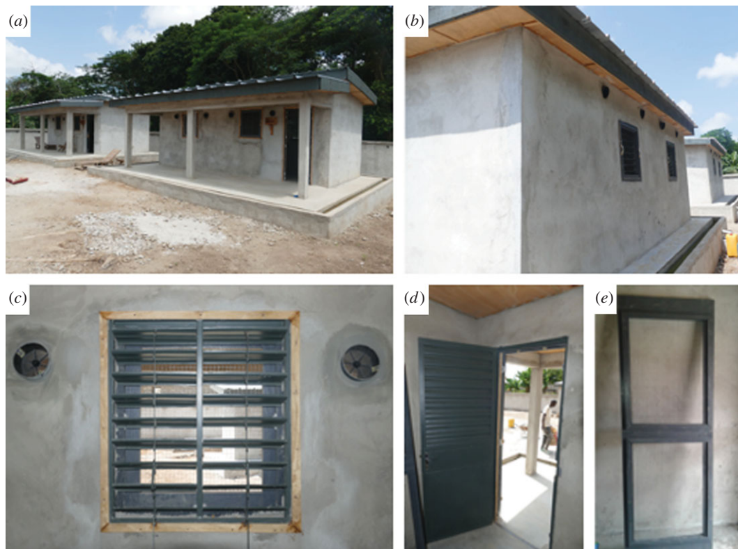
Figure 2. Pictures of the experimental houses. (a) The two experimental houses; (b) back of a house showing EaveTubes; (c) metallic window from the inside; (d) metallic front door; (e) chicken wire frame to put on the front door, which allowed mosquito entry but prevented entry of reptiles and rats when the doors were open.
