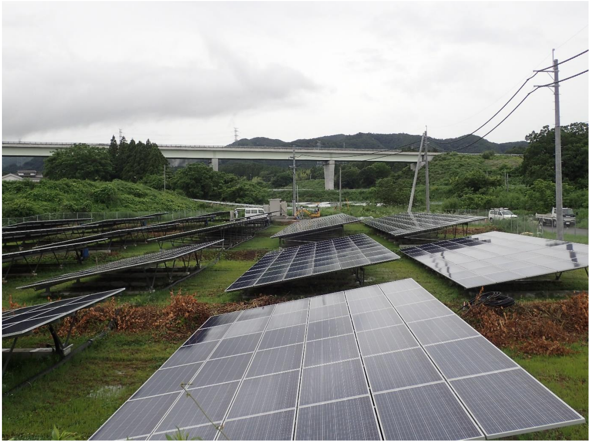
Farmland converted to mega-solar electricity production, Okuma Town (source: author)
