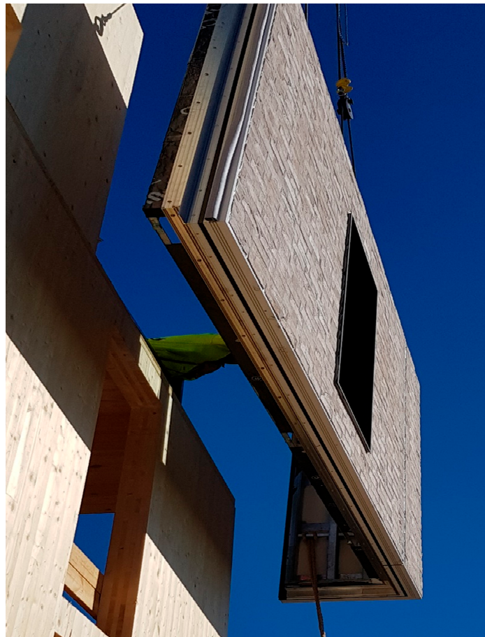
Figure 1. Lifting of a prefabricated façade masonry walling system.
