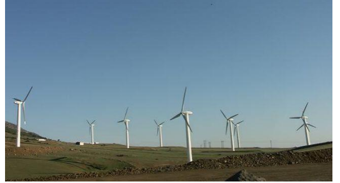
Fig. 4. 90 MW wind farm located in north of Iran
