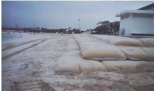
(a) Jumaira Beach Revetment (2003)
