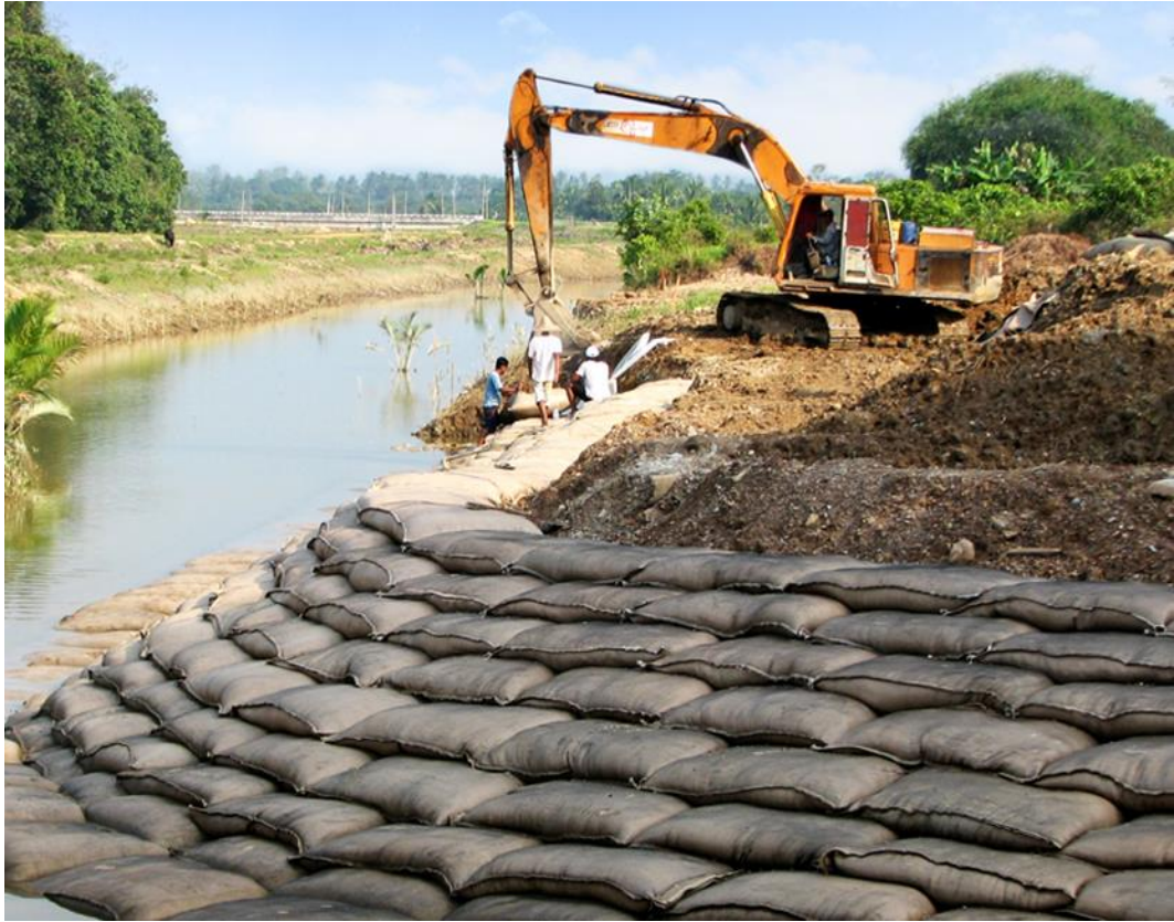
(a) Mechanically installation - Sungai Tenglu River, Johor Malaysia. (TenCate, 2018)
