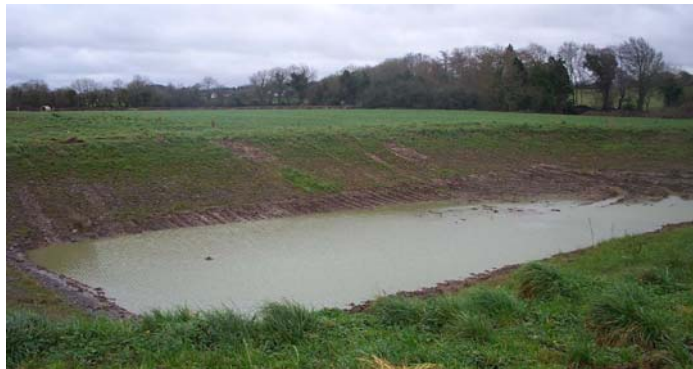
Figure 18: Grange earth-banked tank after emptying (2001)
