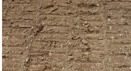
Figure 19: Compacted subsoil liner
