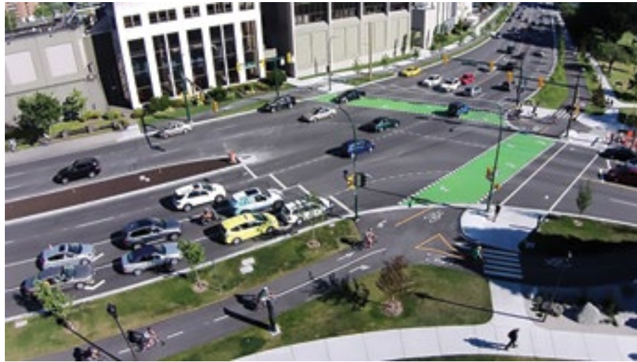
A new protected intersection in Vancouver. (Courtesy of Dylan Passmore)
