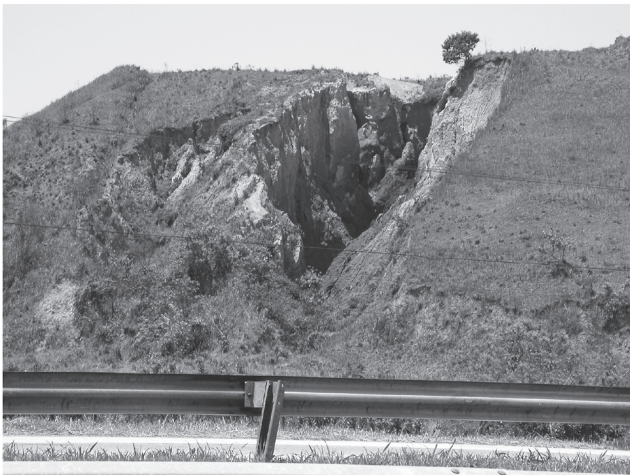
Figure 9 - Deep gully along the state road RJ-122 in the municipality of Cachoeiras de Macacu
