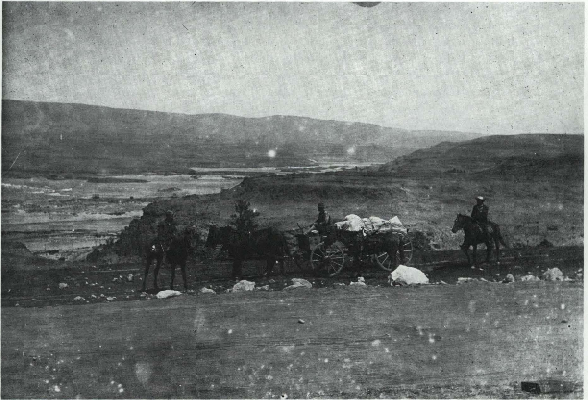
Expedition outfit on road overlooking the Columbia River near The Dalles. Evidence suggests that the photograph is one of Miller's, but it may have been taken in 1901 by another party.
