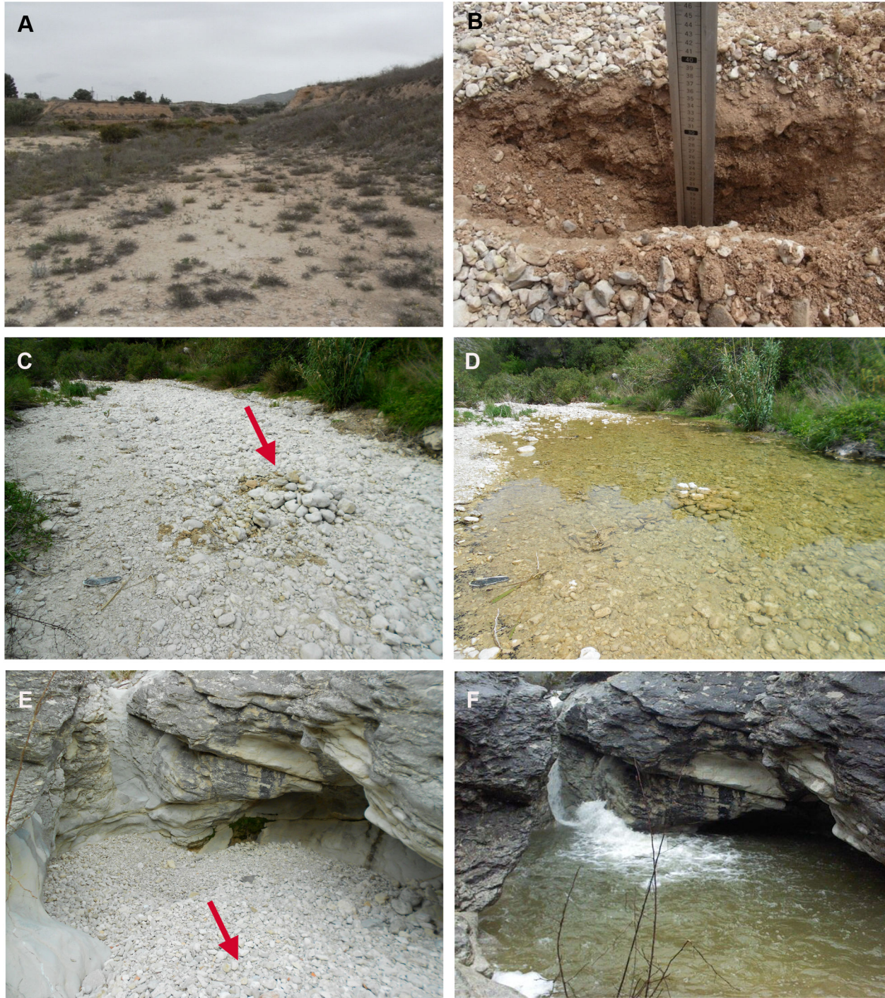
Figure 5. Watercourse with colmated river-bed. (A, B) Rambla de la Torre (Sax, Alicante). Sampled watercourse sections at different moments in time: (C, D) Barranc de la Vall de Gallinera (Subterranean Sampling Device 15); (E, F) Barranc de Famorca (SSD 6).
