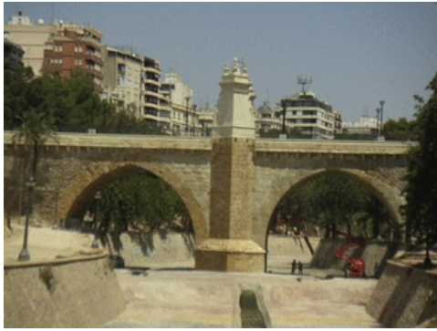
Fig. 1 General view of Elche' Old Bridge, facade N, after restoration (2006).
