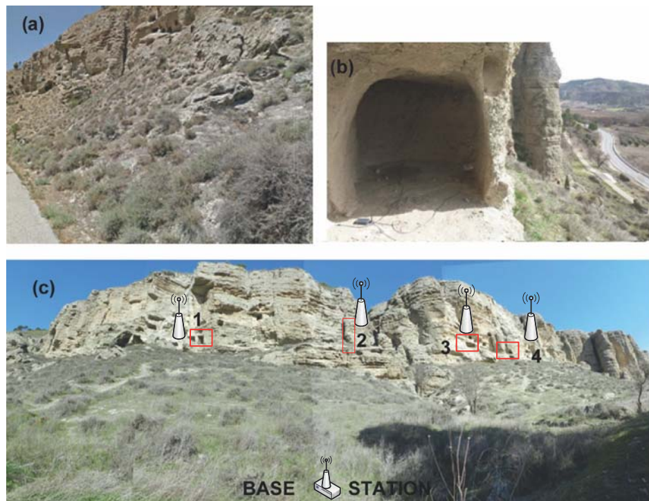
Fig. 8. Network installation at Risco de las Cuevas, Perales de Tajuña, Madrid, Spain: (a) grade on terrain between the base station and caves; (b) sensor installation in mote 3 cave; (c) overview of Risco de las Cuevas showing the positions of the wireless sensor network measuring points.
