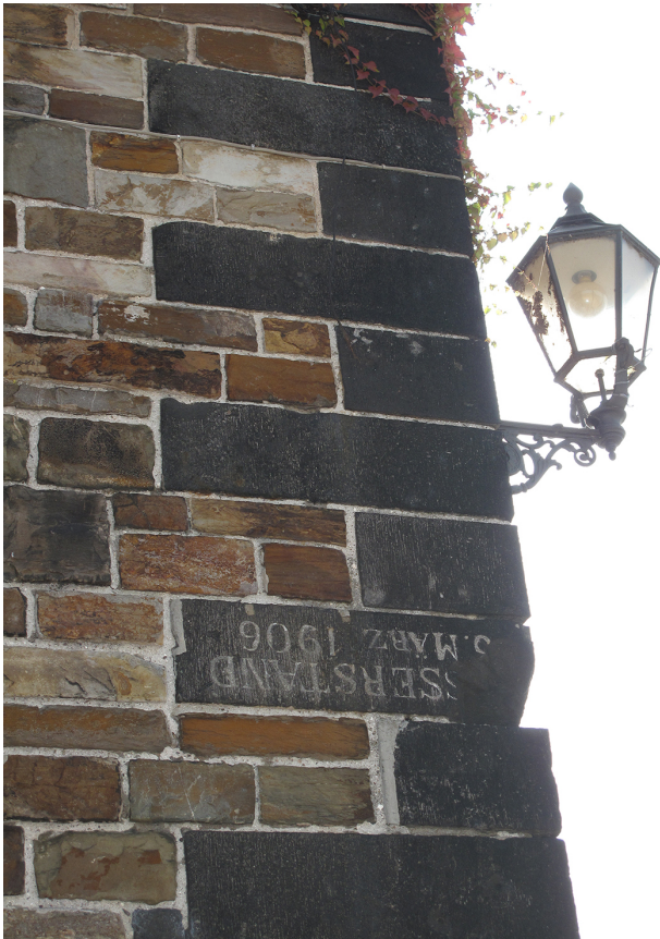
Figure 6. Stone brick with an inscription of the 1906 flood mark of the River Rhine in Koblenz. The block was originally placed on a railway bridge destroyed during World War II and later used for reconstruction of this building (Herget, 2012). This confirms the necessity to work only with the original position of flood marks and to use multiple documentary evidence to reconstruct flood levels.
