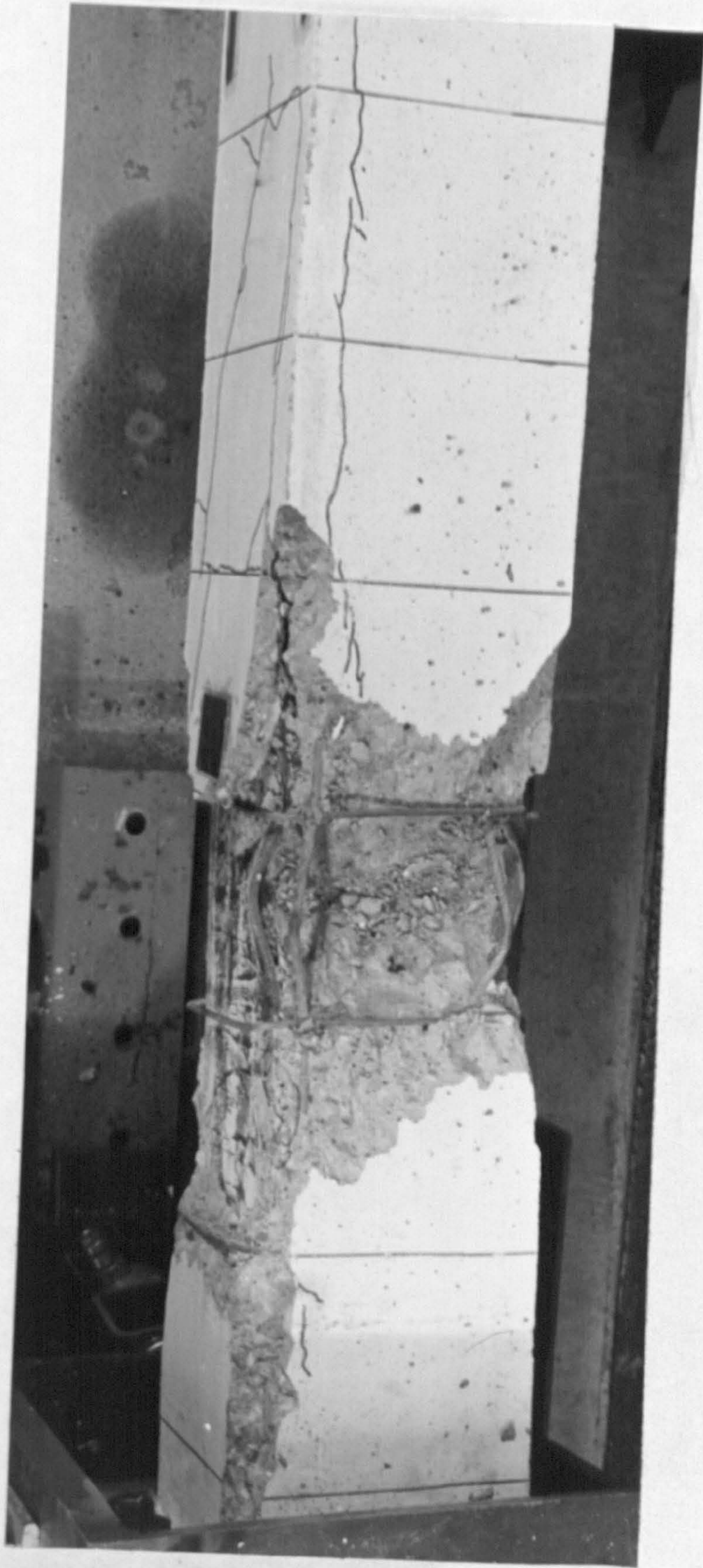
FIG. 6.9 COLUMN RC3 - FAILURE ZONE VIEWED ABOUT MINOR AXIS
