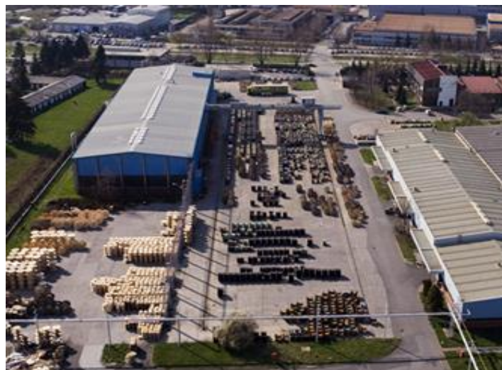
Figure 24. Outside storage area
