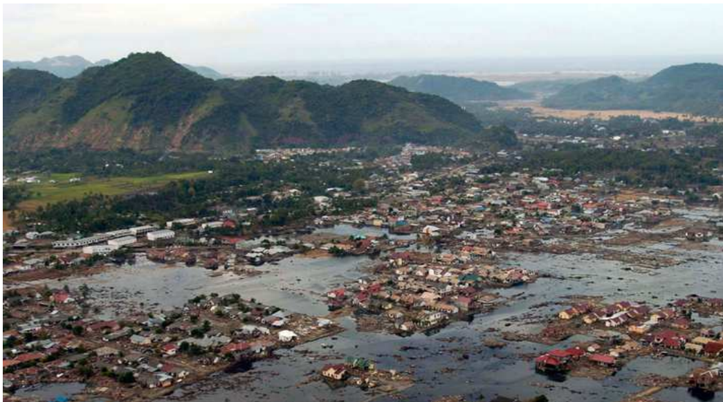
Figure 2.1: A Ruined Village near the Coast of Sumatra in Indonesia after the 2004 tsunami
