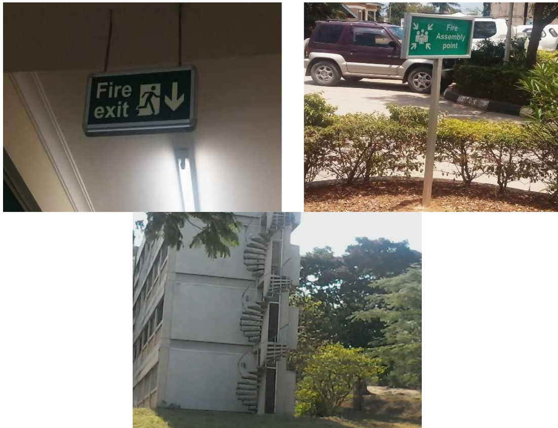
Figure 4.20: Fire Exit Sign (in ODL Tower), Assembly Point at OUT and the Emergency Exit (stairs) on the Staff Residents Building at UDSM
