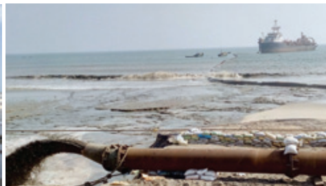
Beach restoration process by dredging
