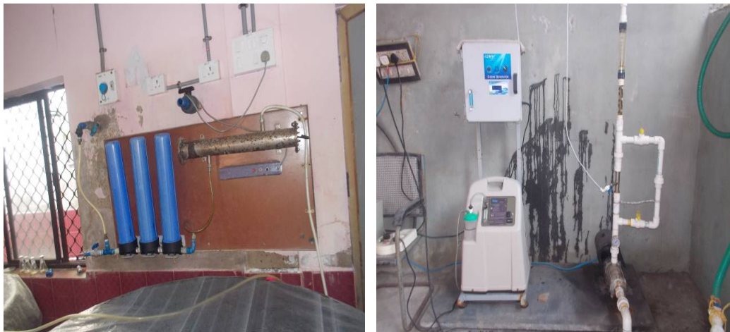
Fig. 3. Disinfection by Ultraviolet radiation and Ozone treatment
