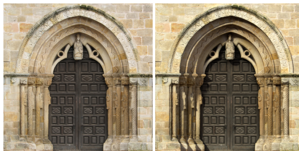
Figure 1: Portada de la Oliva, Asturias, Spain. Orthoimages of the same object generated from photographs taken either in cloudy conditions (left) or under direct sunlight (right).
