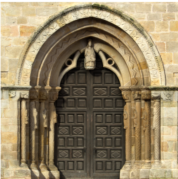
Figure 10: Final orthoimage, made by composition of layers with alternative position for the sun w.r.t Fig.3.
