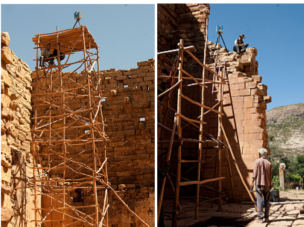
Figure 2: Scanning on scaffolding (left) and on top of the wall (right) using the IMAGER 5006 from Zoller + Fröhlich
