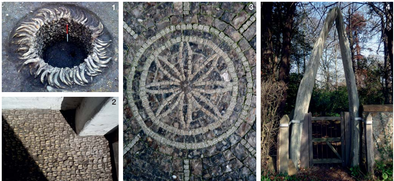
Fig 3.5 The structural use of animal bone. (1) Horn-core well lining at Prescott Street, London. Details of floors at (2) Wantage, Oxon, using phalanges, and (3) West Dean, W Sussex, using horse teeth. (4) Whale jaw arch, Chideock, Dorset. [(1) Photo LP Archaeology, (2) photo P Wilkinson, (3) photo P Baker, (4) photo P Baker]
