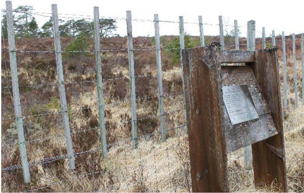
Figure 5-9: Tfl's first deer enclosure showing retrofitted wooden slats to prevent grouse injury. The plaque commemorates the opening of the enclosure in 1990, 25/11/16.
