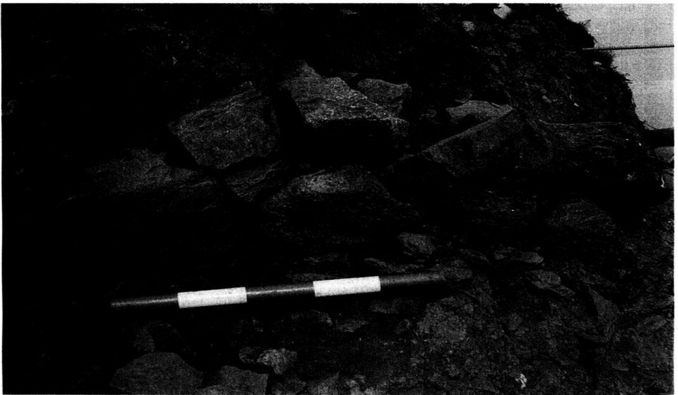
Fig. 9. Area 2, retaining wall (281), view north-east, scale 0.5m.
