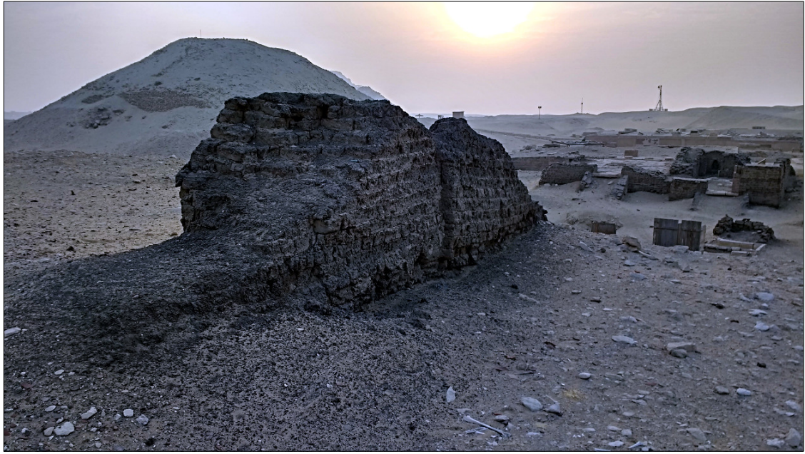
Figure 5.6. The possible southern wall of the Serapeum Way, perpendicular to the Anubieion western wall. The pyramid of Teti is visible in the background with various structures of the Teti north cemetery visible to the right of the image (photo author).
