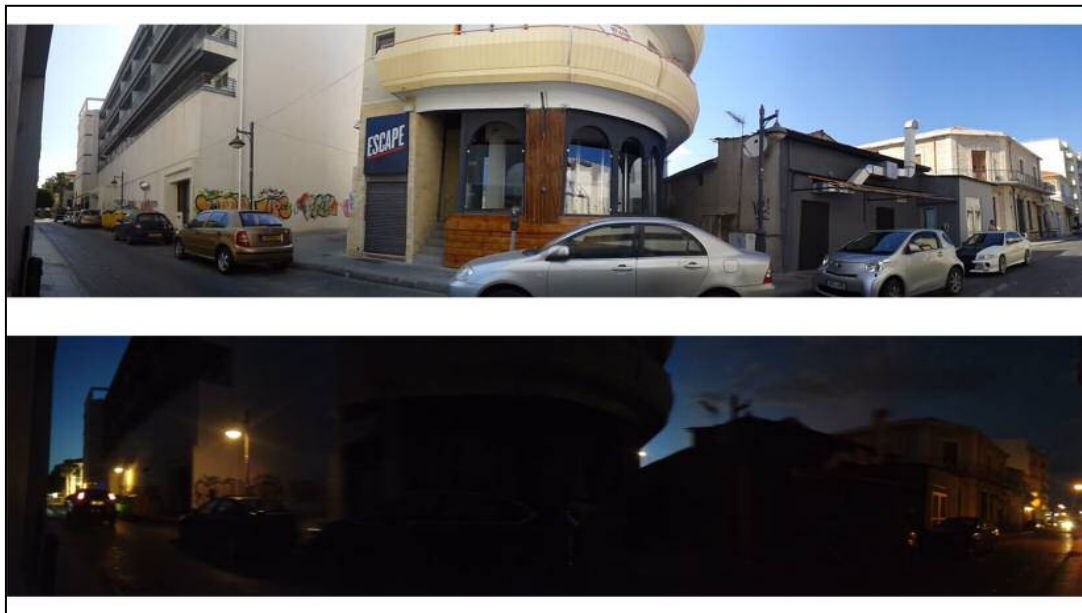
Figure 6.15 Poor night-time lighting around Heroon Square xiii
