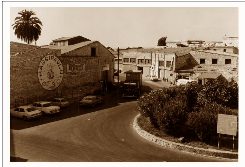
Figure 3.11 Warehouses marking Limassol's urban landscape xiii
