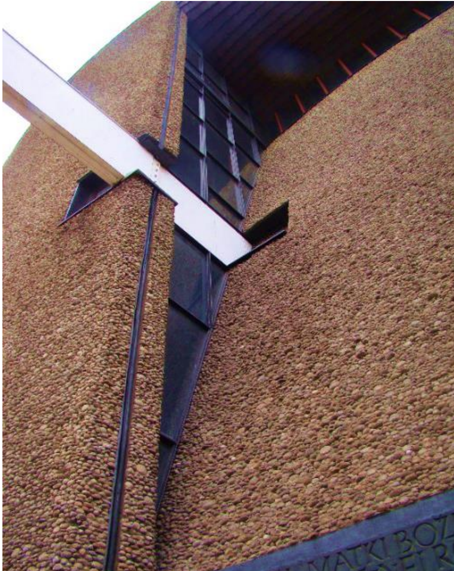
Fig. 5.39 Elevation of the church-Concrete with river-bed rocks as aggregate; Author's own photo
