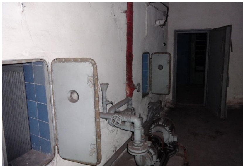
Fig 5.26 Basement of Kino Switowid; Author's own photo
