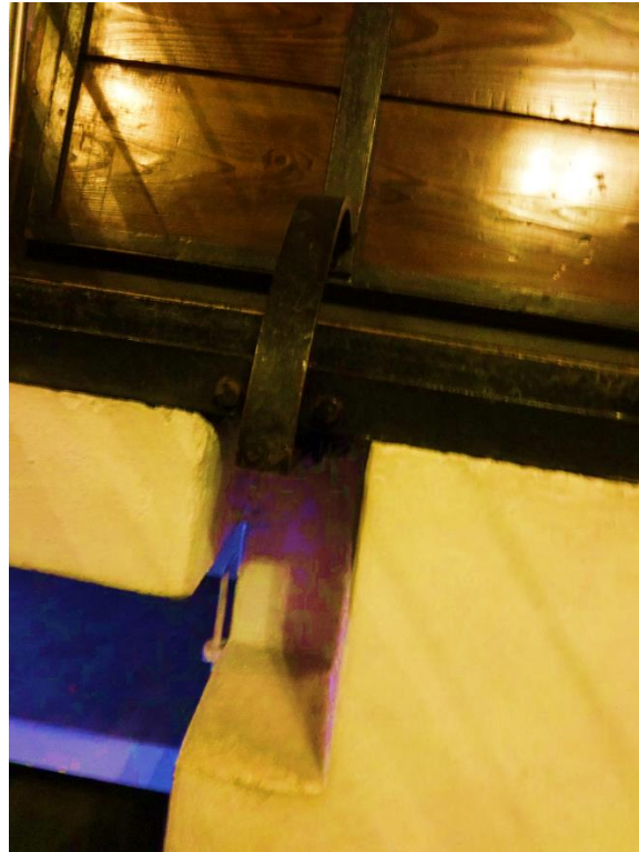
Fig. 5.64 The hinges of the doorway leading to the crypt in St. Maximilian, Own archive
