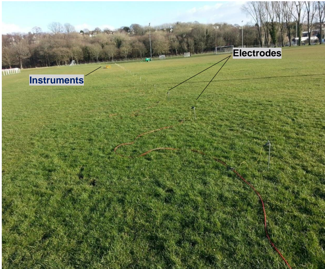
Figure 3.15: The soil resistivity set up at the earthing system facility at Llanrumney site.
