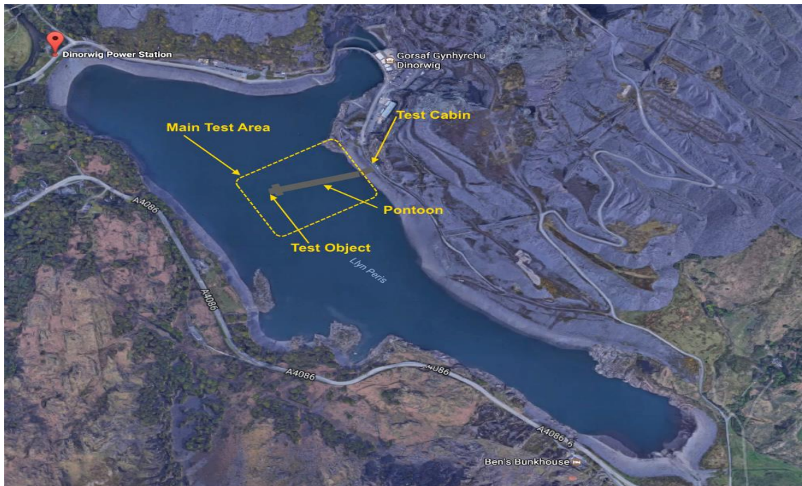
Figure 3.8: Aerial view of the lower reservoir at the Dinorwig power station and test area.
