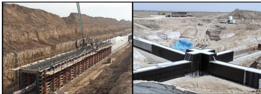
Figure 7.7: Underground concrete services tunnel
