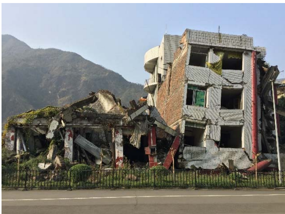
Figure 4: Example of soft-storey phenomenon in a building in Beichuan
