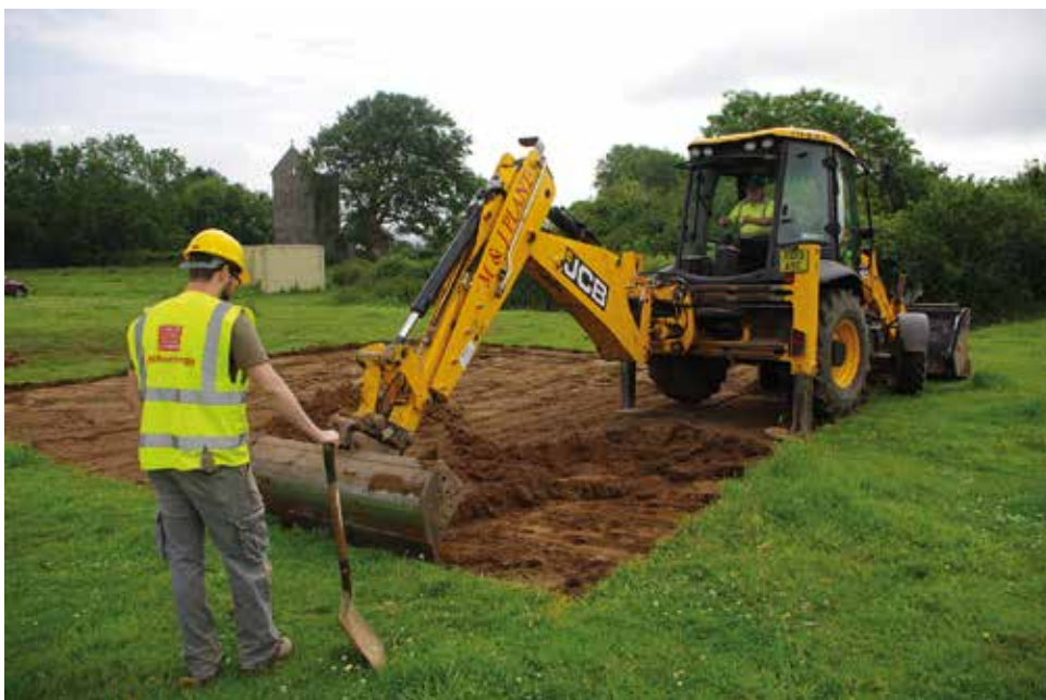
Fig. 4.2. Photo showing machine stripping of topsoil and relict ploughsoil over the area of Trench 5A
