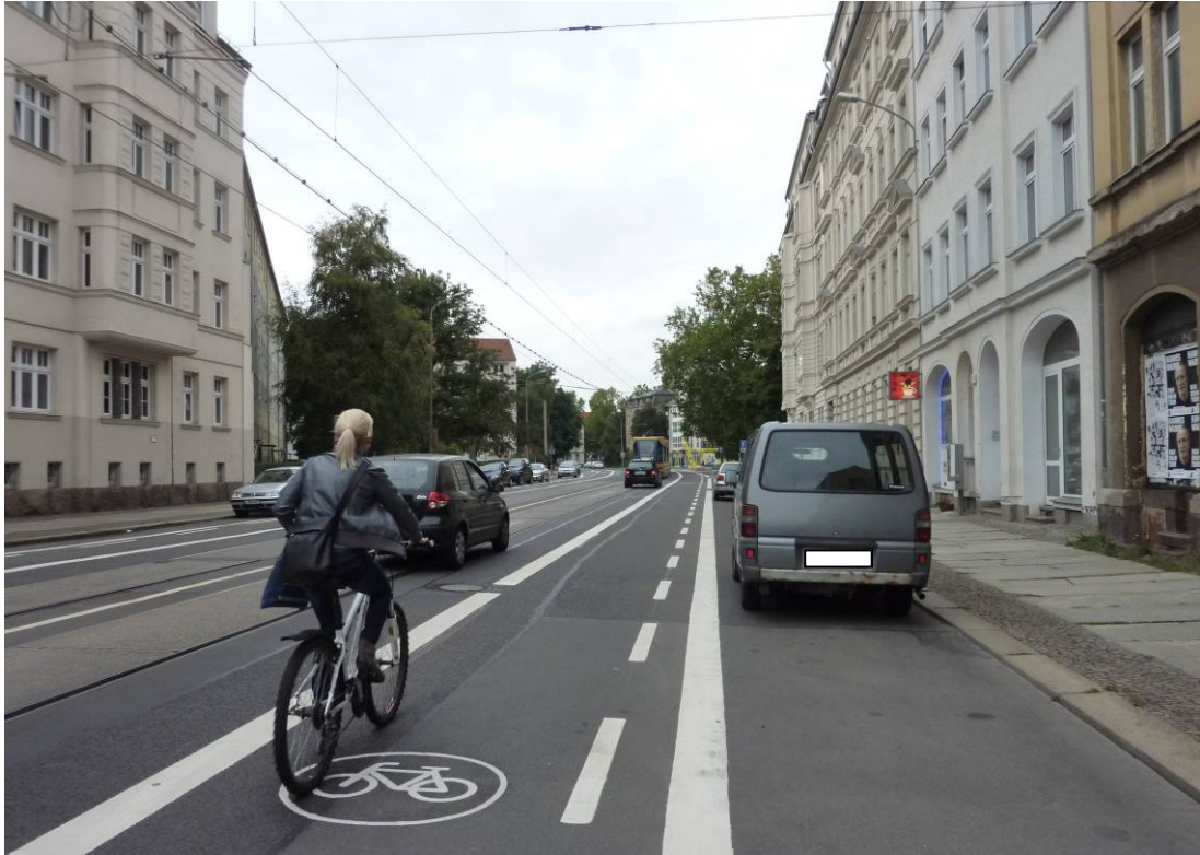
Figure 6. 2: New marking of the Georg-Schumann-Street, now the street has only one lane per direction, a separate bicycle path and parking off the pavement
