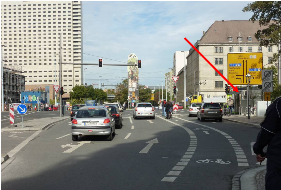
Figure 7. 4: View from the entrance of the car park towards the measuring station (arrow)
