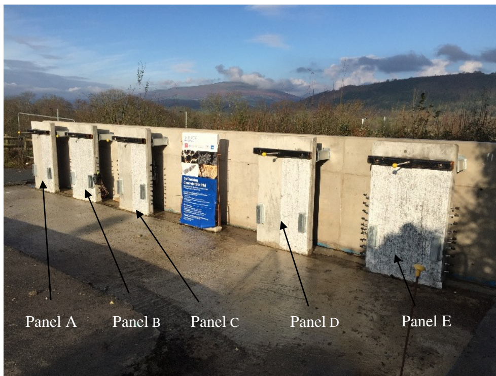
Figure 7: Site trial panels after initial loading
