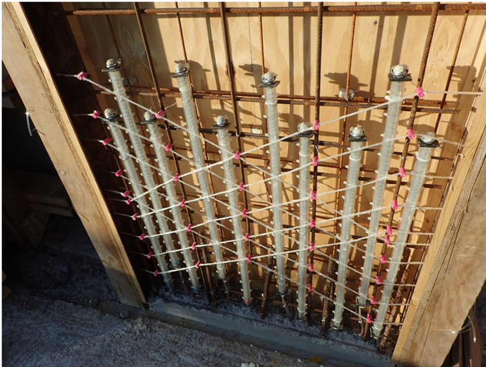
Figure 6: Shape memory polymer tendons and vascular network setup before casting concrete
