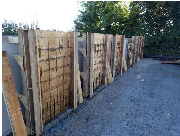
Figure 4: Formwork and reinforcement setup for trial panels
