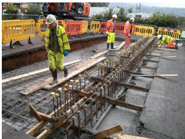
Figure 3: Casting of concrete base slab and kickers
