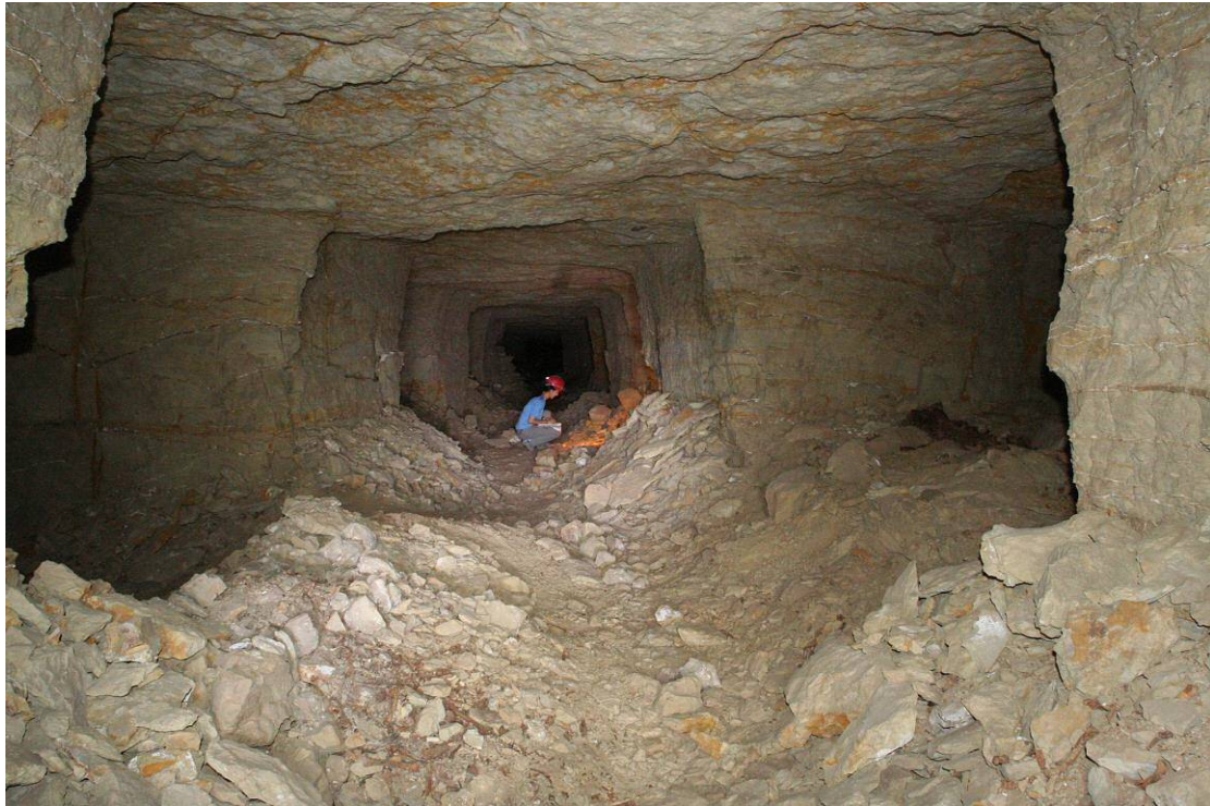
Figure 4. Looking along the axial aisle of the Dog Catacomb. The effects of scabbing can be seen at the foot of the walls. (Photo: P.T. Nicholson).
