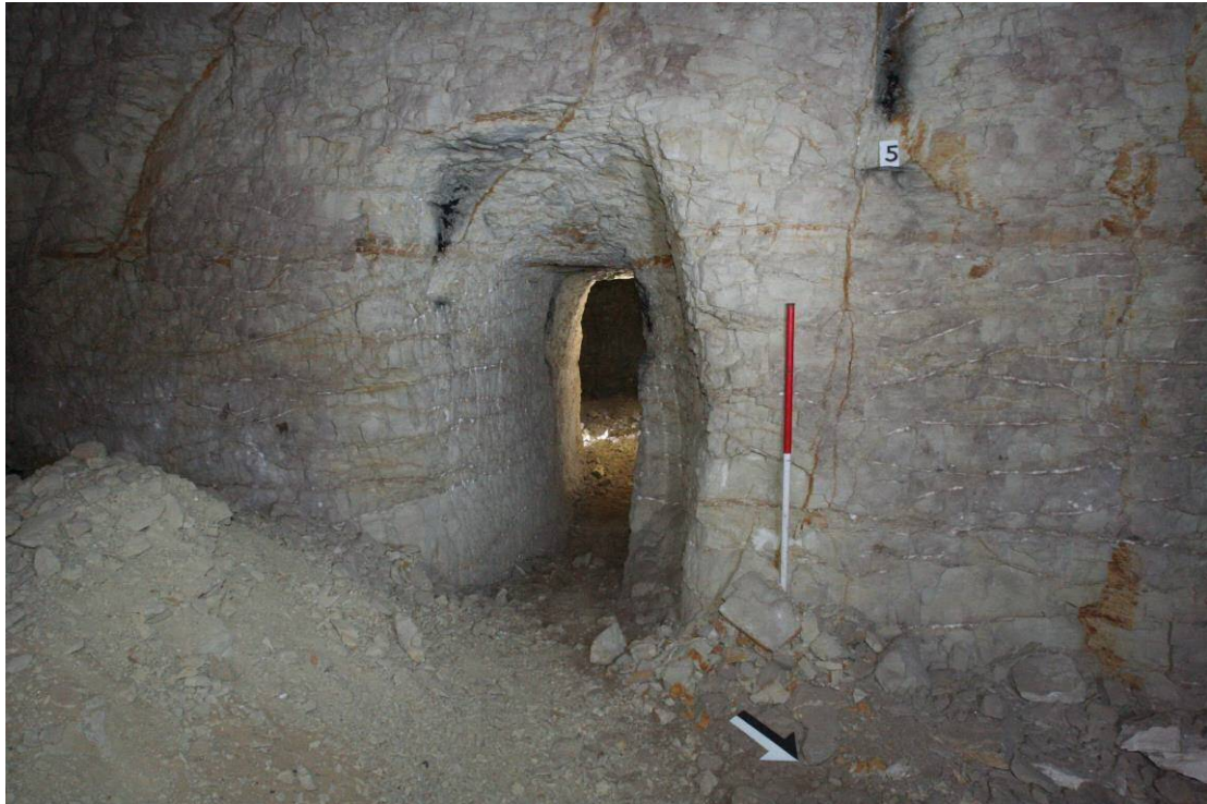
Figure 12. A secondary doorway cut between galleries 5 and 6. As well as having rubble from its cutting nearby it also has the characteristic lamp niches outside it and along its length (see figure 10). (Photo: P.T. Nicholson).
